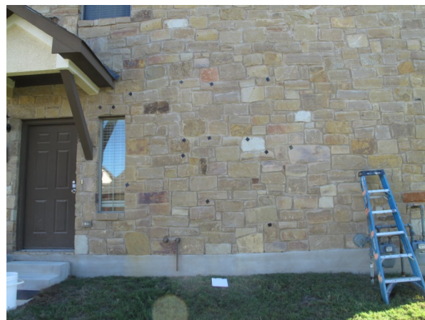
Figure 9: Overview of typical survey area at stone masonry veneer.
